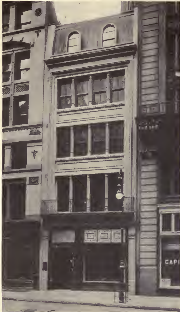
EXTERIOR OF BUILDING AFTER REMODELING
